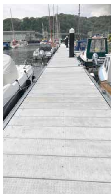
These are light grey stipple effect GRC pontoons at Fowey
