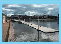
access, which had become precarious. With the site drying out on every tide, the new pontoon, moored on piles, required grounding brackets. The tidal variation also meant that a specially designed 17m x 3.5m gangway was necessary for the rowers to access the pontoon, and safely carry their boats to the water for launching at all states of the tide.
