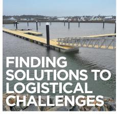
With demand exceeding supply for berthing facilities in Stornoway, we installed our standard GRP mini mesh decked marina pontoons, with excellent anti slip properties, to provide the much-needed additional marina pontoon berths.
