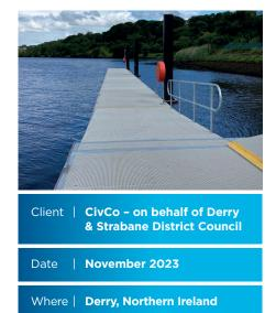
"Considerably longer than what would be required on inland rowing facilities, the three-gangway set-up was required to allow the rowing boats to be carried parallel to the line of the pontoons."
